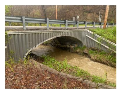
Figure 3. Metal Culvert
