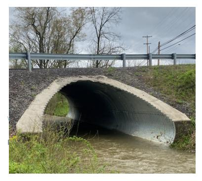
Figure 4. Metal Culvert
